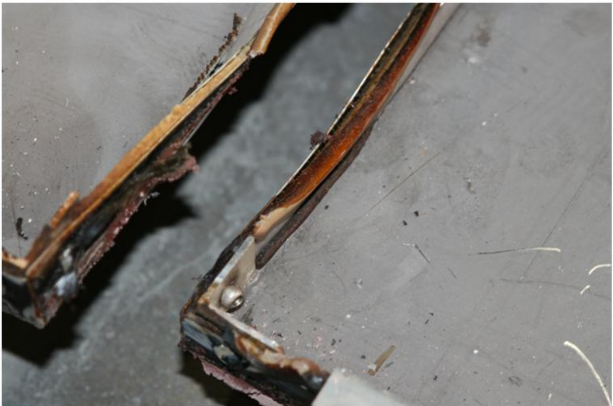
Figure B-6. Backside of Panel Following the Test.
