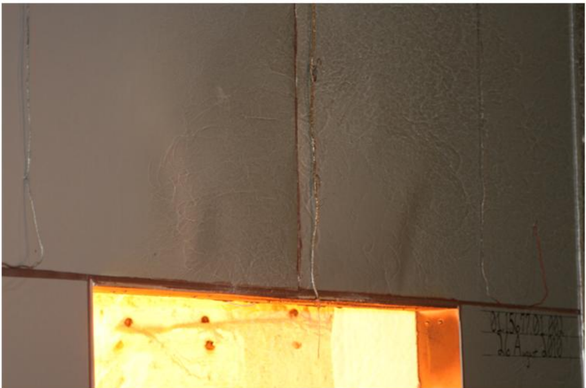
Figure B-2. Initial Deflection above Window.
